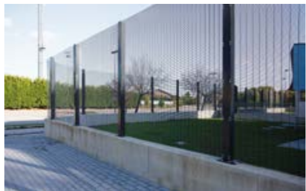
Omega post with 90x4 or 120x4 mm cover plate
