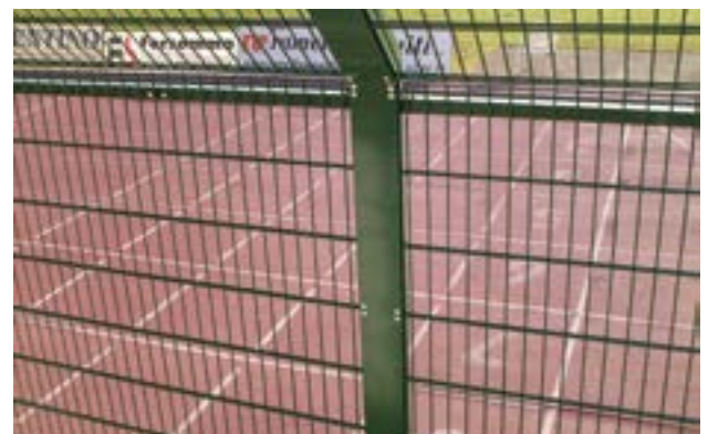
Omega post 120x60x30x3 mm section
