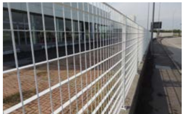
49x25x11 mm C-shaped welded post
